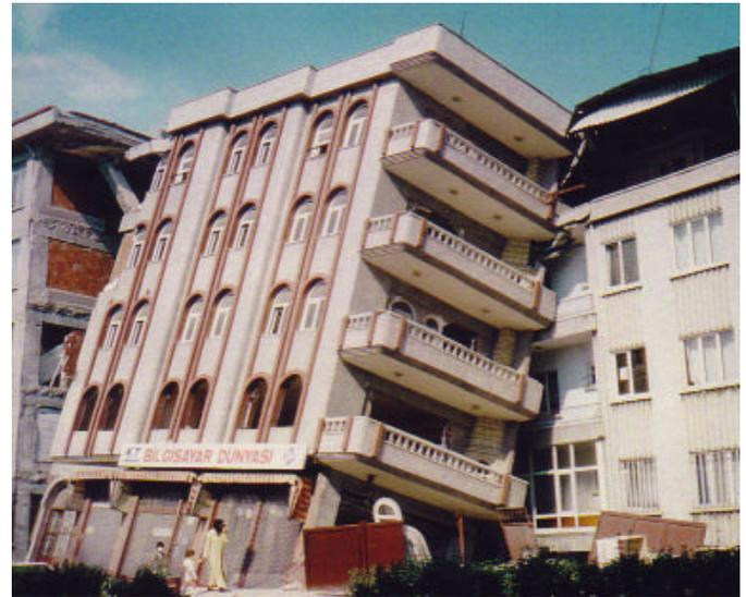
*Fig.11. Liquefaction induced foundation failure in Adapazari during the Kocaeli earthquake*
