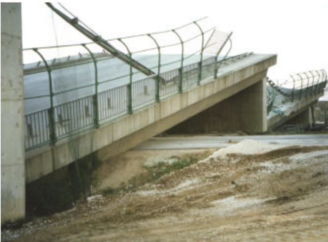
*Fig.13. Unseating of bridge decks from piers of the Arifiye Bridge traversed by surface fault*
