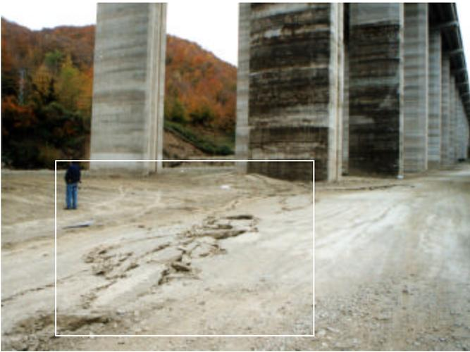
*Fig.12. Piers of Trans-European-Motorway (TEM) traversed by surface fault rupture, Kaynasli, Düzce*
