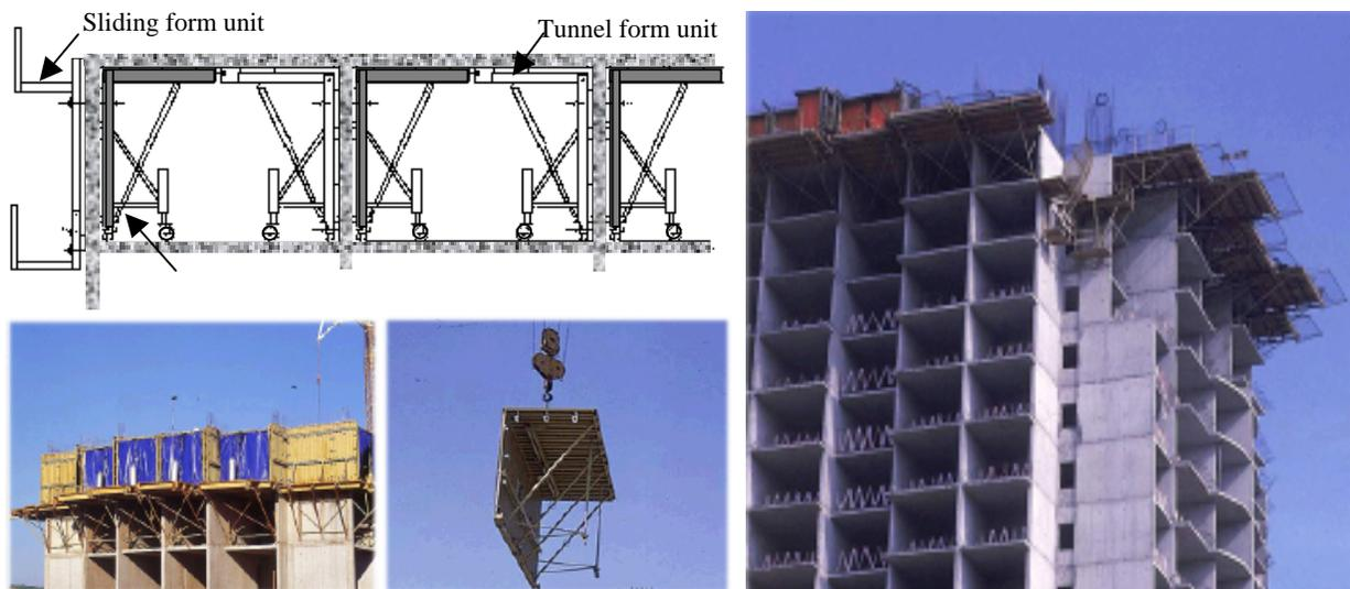
Figure 1. Typical implementation of tunnel form construction system
