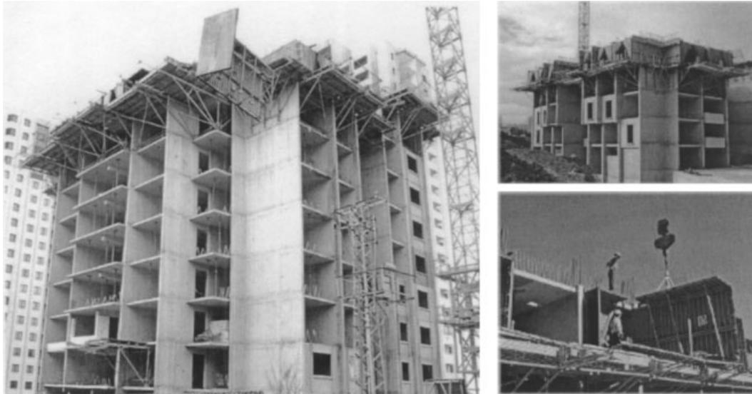
Figure 1. Tunnel form technique and construction system.
