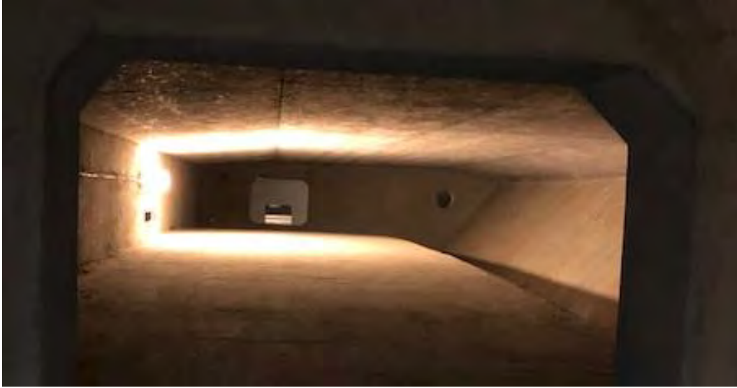
Figure 2-9: Interior photograph of arch merge region
