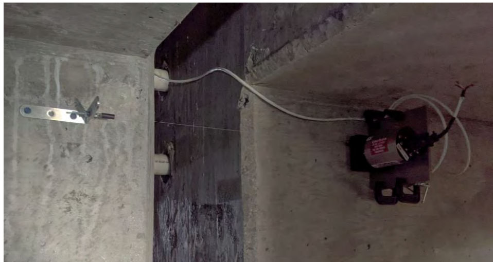
Figure 3-13: Example of potentiometer installed at Hinge 1
