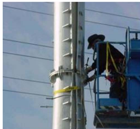
Fig. 1. Constructive details of steel jacketing and field application of retrofitting.
