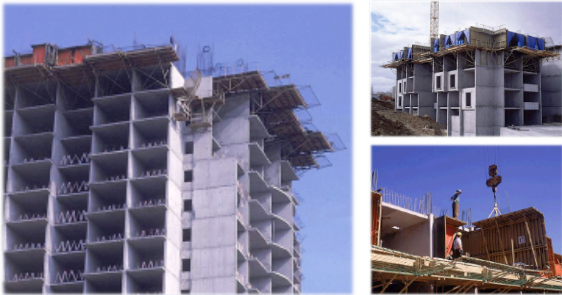
Figure 1. Tunnel form construction technique and its special formwork system
