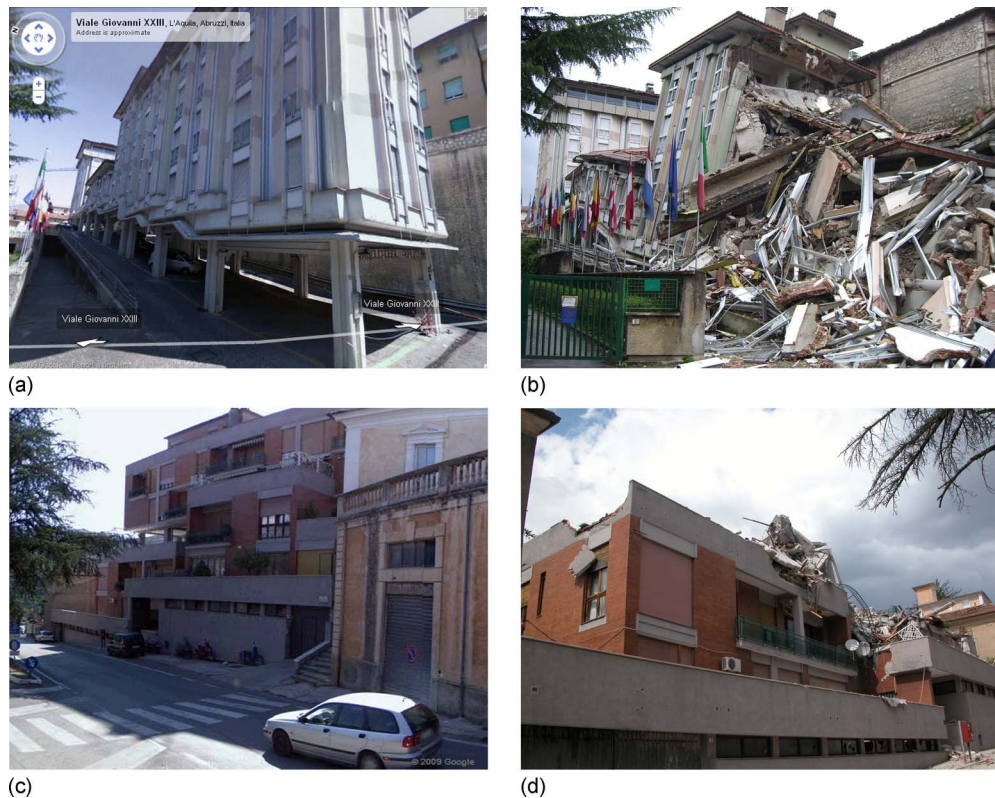
Figure 4. (a) Condition of Hotel Duca Degli Abruzzi in L'Aquila before the earthquake as obtained from Google Maps Street View and (b) the post-earthquake condition observed from the ground. It is possible to observe the presence of a significant irregularity in elevation between the ground and the first floor. (c) Before and (d) after earthquake condition of another collapsed building (irregularity in elevation at intermediate floor) in L'Aquila assessed by similar methods.
