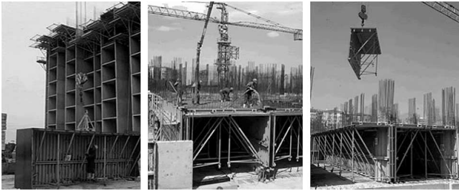
Fig. 1. Tunnel form construction and its formwork system.
