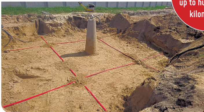
Measurement of a ground vertical displacements – R&D field
