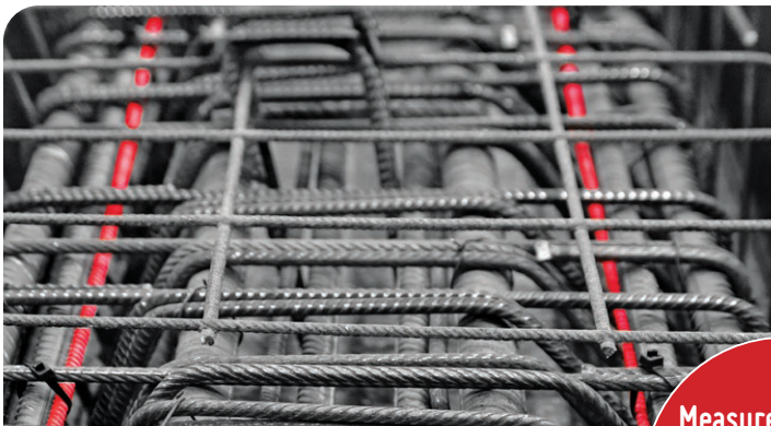
Prestressed concrete beam with EpsilonRebar
