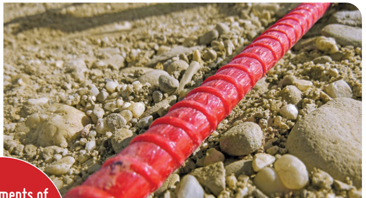
Road embankment with EpsilonRebar
