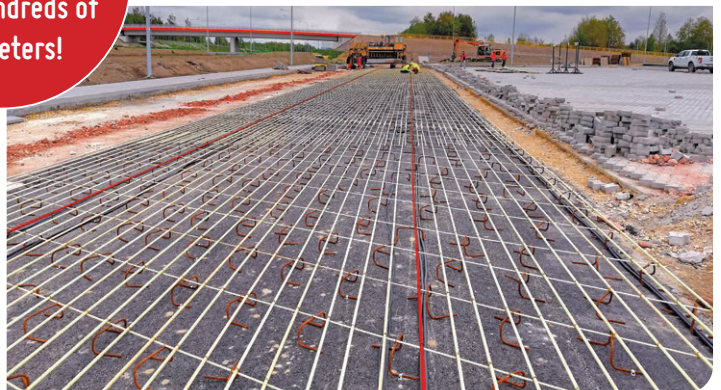
Application of EpsilonRebar in a smart concrete highway
