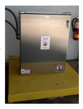
The digital tri-axial seismic sensor measures earthquake intensity in "g" force, and stores Peak Grou nd Acceleration values (PGA) in memory for future engineering analysis. Filtering devices make it immune to industrial vibrations such as heavy equipment etc.
