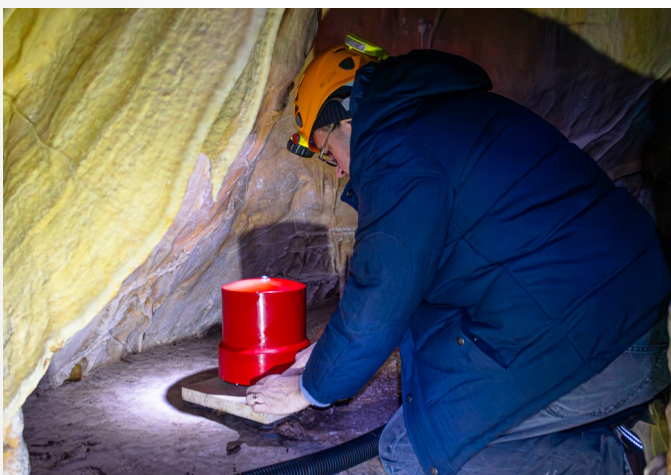
an underground SS08 installation in central-Italy
