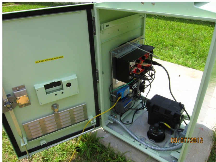
Figure 2. Seismic substation example with Wi-LAN telemetry hardware. Station is powered by grid. A single sealed lead-acid battery is used as a backup power. (Photo source: USGS)
