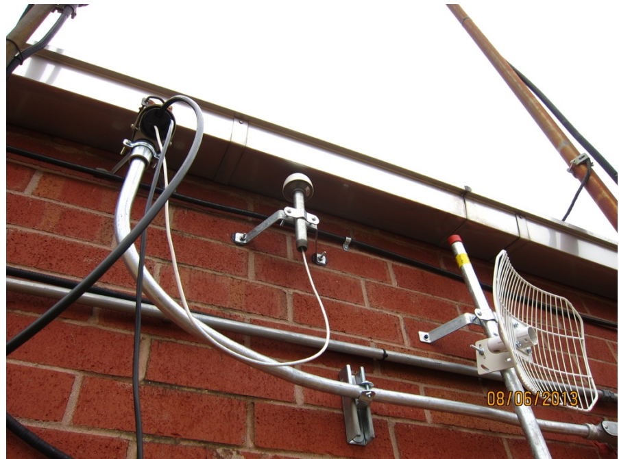
Figure 2. Seismic base station example with Wi-LAN telemetry hardware. Station is powered by grid. (Photo source: USGS)
